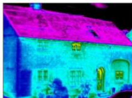
Grade B, old refurbished property
